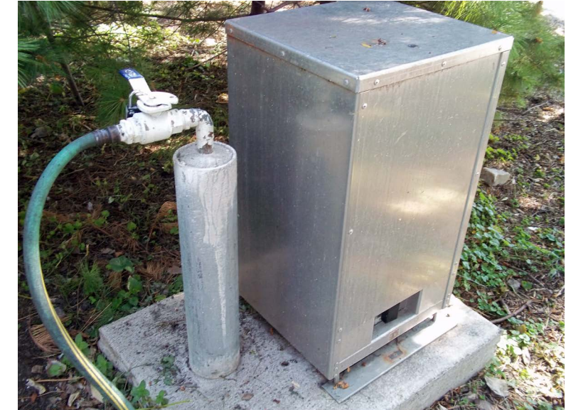
Fig 85: Water source that NeighborSpace will install at the garden.
